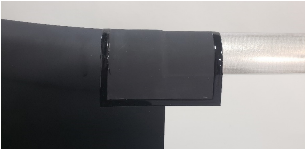
Figure 4 ~ Completed Polyurethane Tape Installation – Inboard Abrasion Strip Joint
